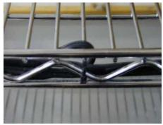
Figure 5: Tie wrapping wires to the inside of the shelving unit
